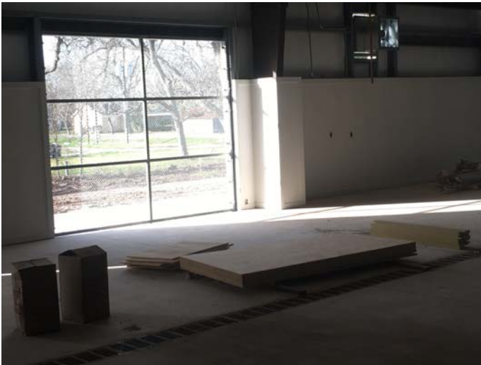
1. Installation of bird screens at sliding doors
