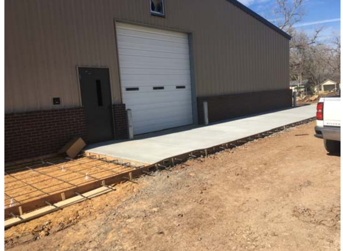
4. Concrete walk at front elevation
