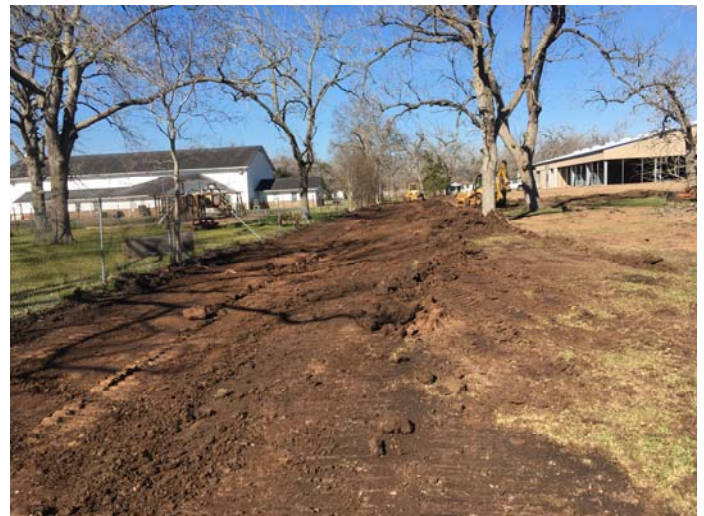
6. Excavation of drainage swale on north property line
