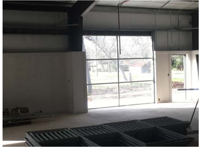
2. Installation of bird screens at sliding doors
