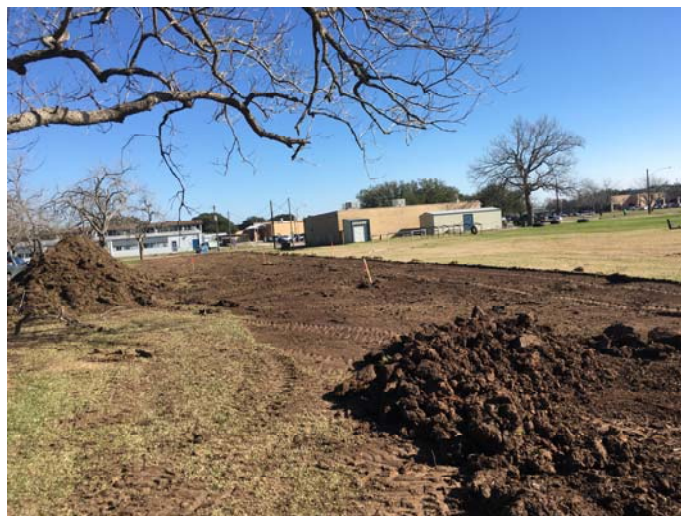
5. Excavation of drainage swale on west property line
