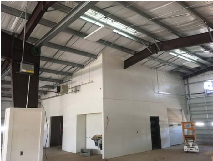
3. Painting of finish carpentry above restrooms
