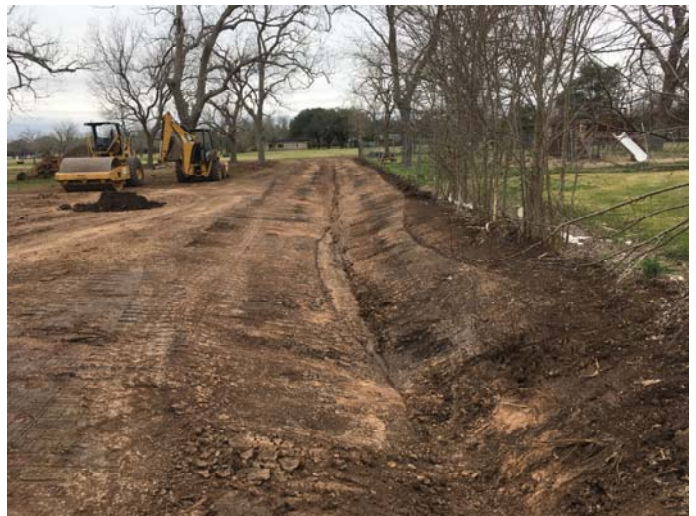
8. Drainage swale on north property line
