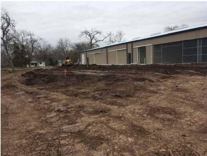
9. Placement of fill for final grade
